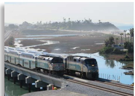
The more than 70-year-old existing wooden trestle bridge was replaced with a modern, double-track bridge. Its wider spans help improve tidal flow in the lagoon.
