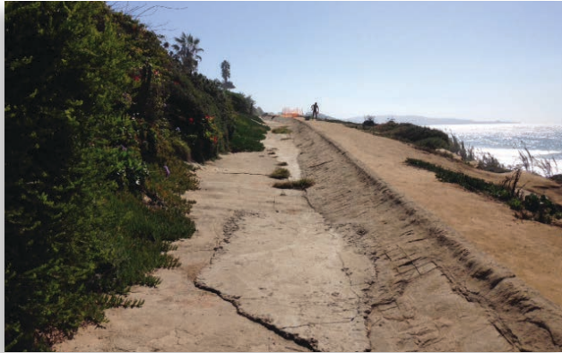
7th Street Drain to be reconstructed
