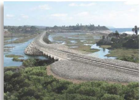
*The more than 70-year-old existing wooden trestle bridge will be replaced with a modern, double-track bridge. Its wider spans will help improve tidal flow in the lagoon.*
