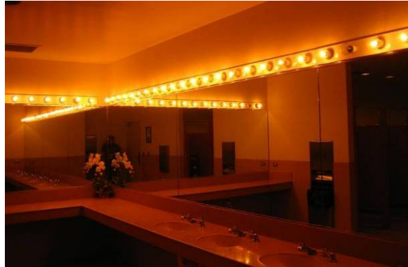
Figure 30 Restroom with 42 Lamps around Mirrors
