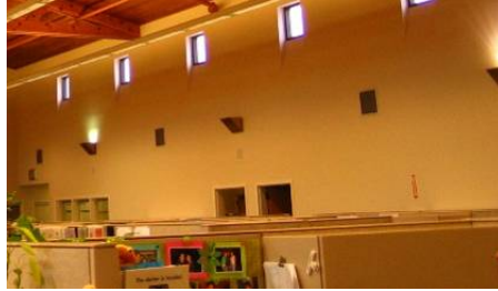
Figure 375 Wall-washer light
