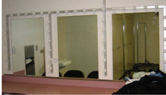
Figure 32 Incandescent Lights in Dressing Room
