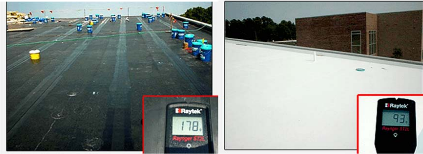
Figure 11 Before and After Cool Roof
