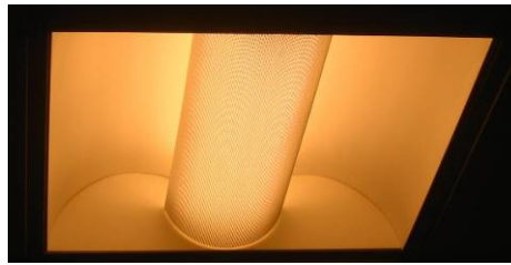
Figure 2 CF 40 Fixture with 26W Lamps
