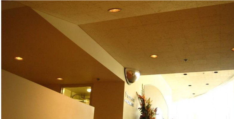
Figure 27 Recessed Can Lights with Par 38 Lamps
