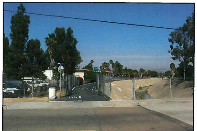
Looking east along bike path from Juniper St.
