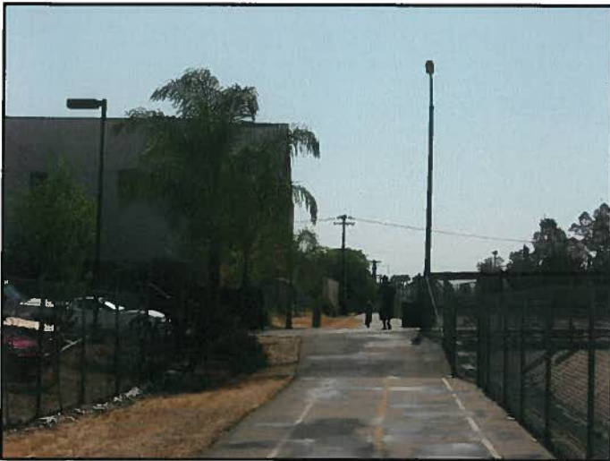
Looking west along bike path at Date Street Bridge (bike path transitions from north side to south side of the channel at Date St.)
