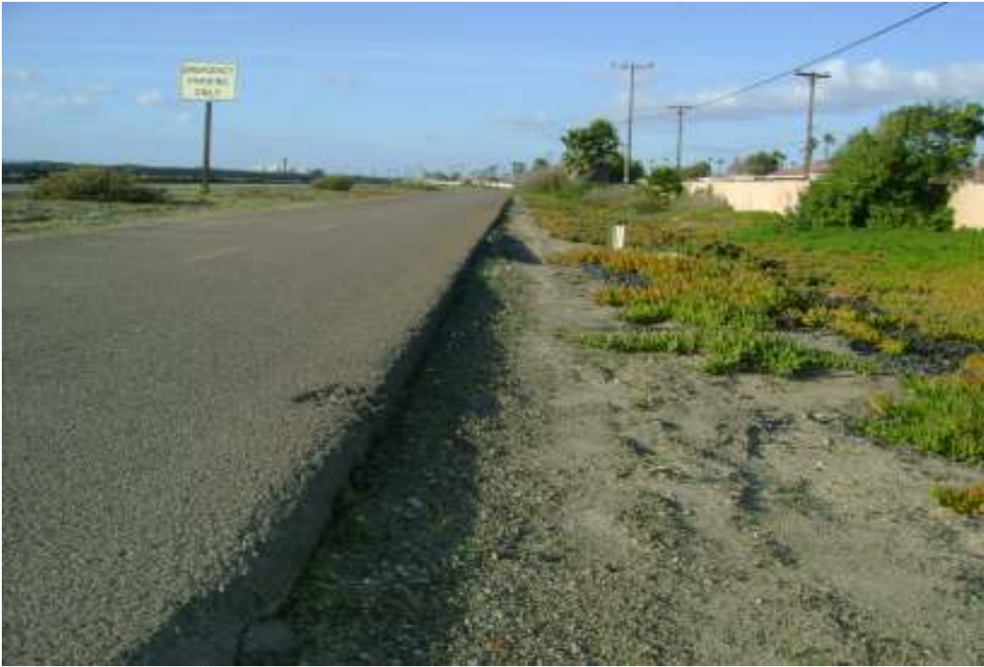
Photo A - Located in Segment 1
