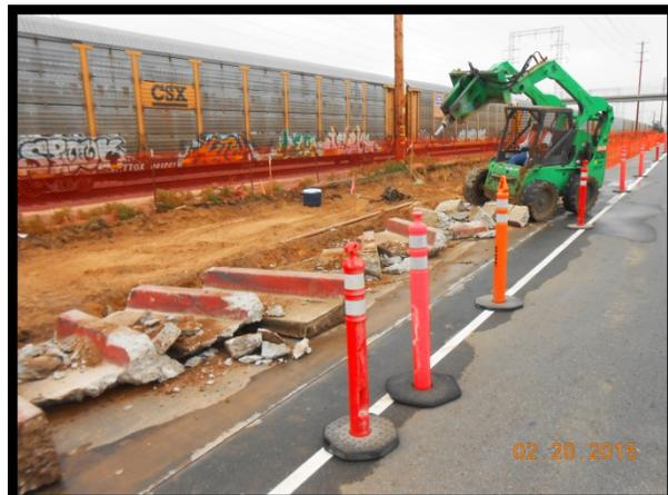
Sawcut AC/ Demo Curb &amp; Gutter 10+00 to 12+80
