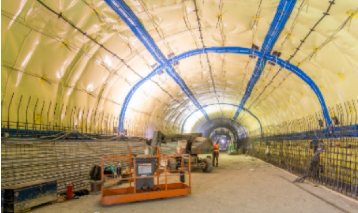
Figure 6.9. Installed PVC Waterproofing
