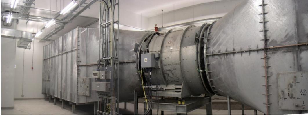
**Figure 8.5. Typical Tunnel Ventilation Fan with Duct Transitions and Attenuators**
