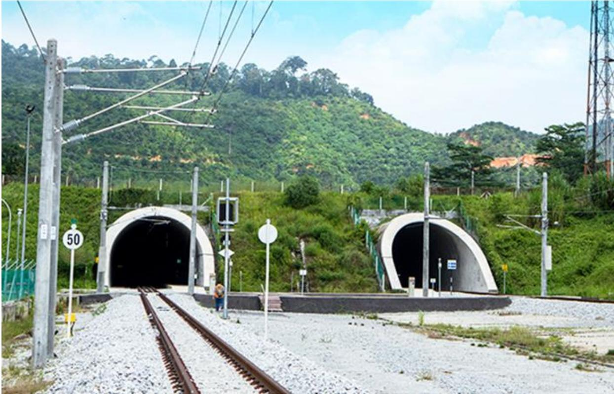
Figure 8.4. Tunnel Portal Showing Emergency Assembly Area, Trackway Crosswalks
