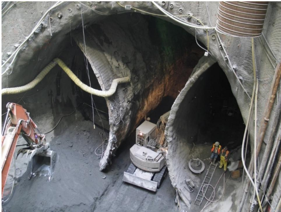
Figure 6.8. Typical SEM Tunnel Construction Sequence and Support
