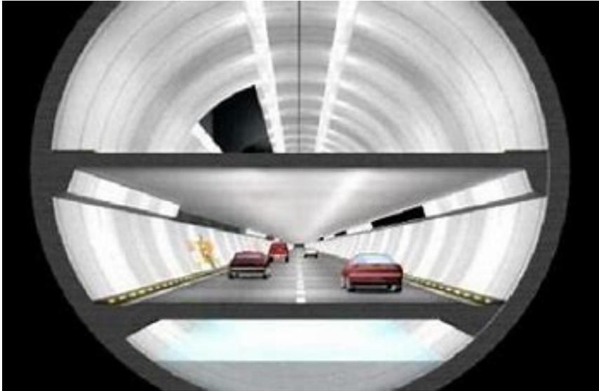
Figure 12.2. The SMART Tunnel in Malaysia: Road tunnel combined with storm drain
