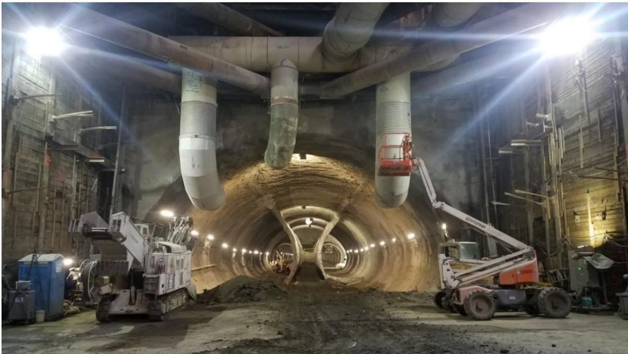
**Figure 6.6. SEM Tunnel Showing Pocket Excavation, Regional Connector, Los Angeles**
