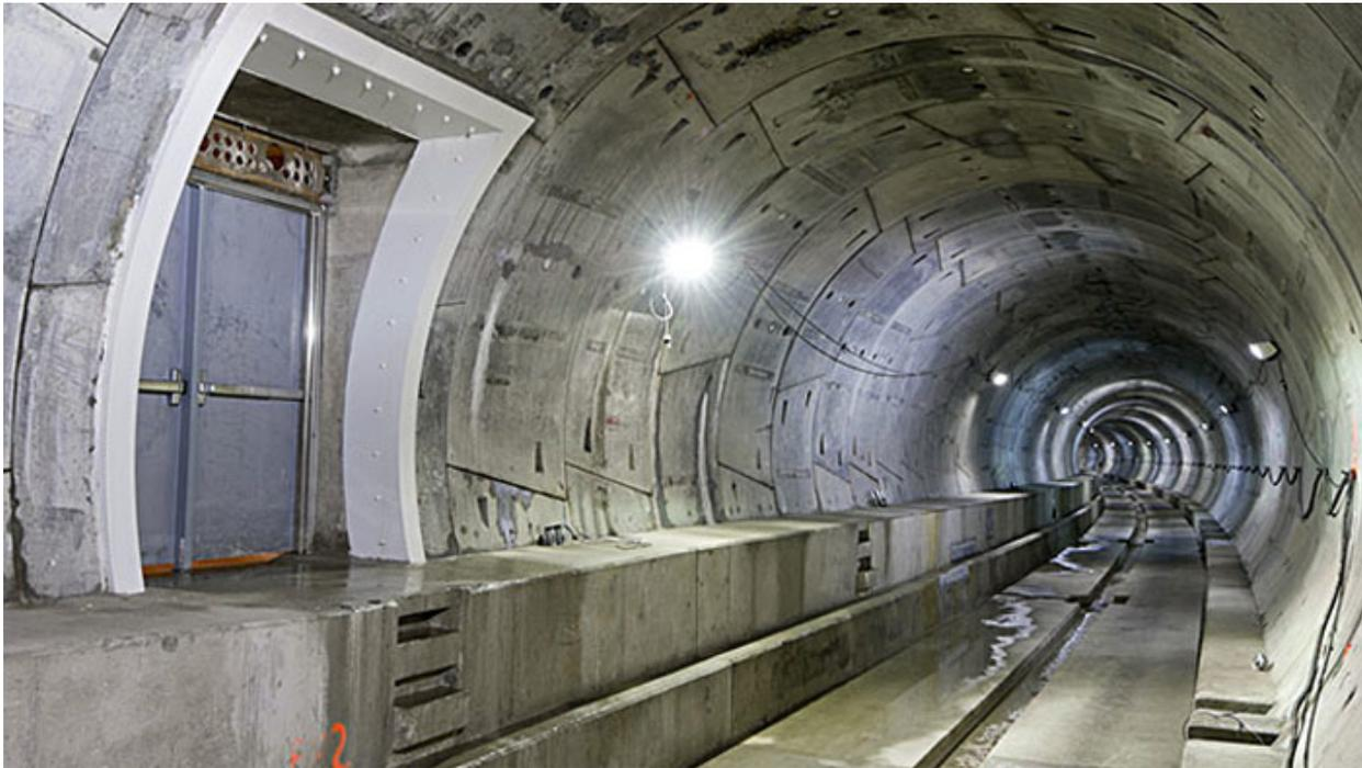
**Figure 6.1. View of a Cross-Passage Access from a Tunnel**
