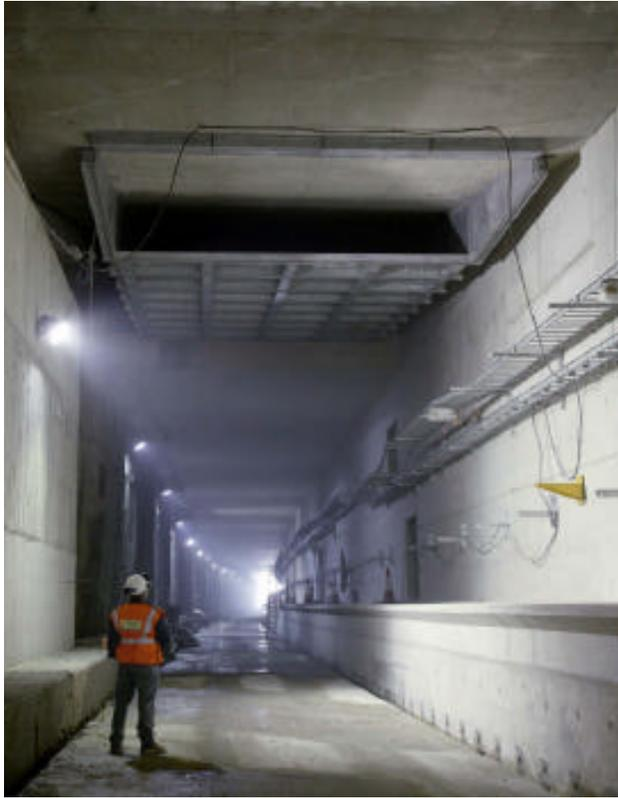
Figure 8.8. Photo of Nozzle in Tunnel
