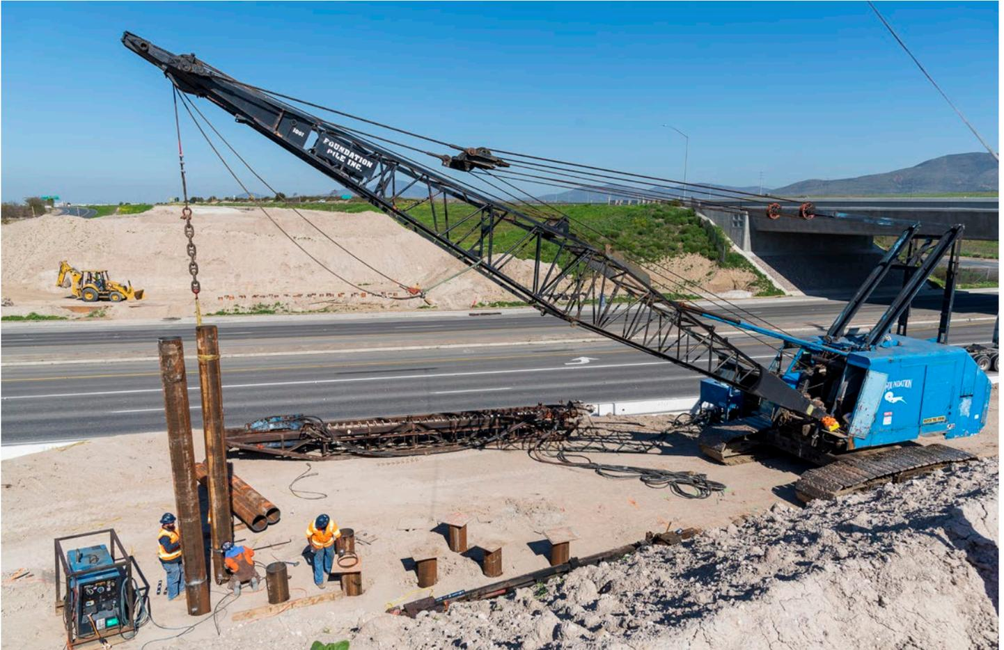
Caltrans and SANDAG crews install piles just south of Otay Mesa Road to support the new SR 11 connector ramp to SR 125.
