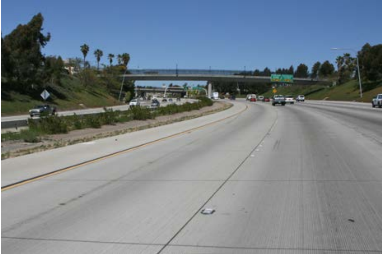
Existing Conditions: View heading northbound on SR-15 approaching Landis Street Bridge
