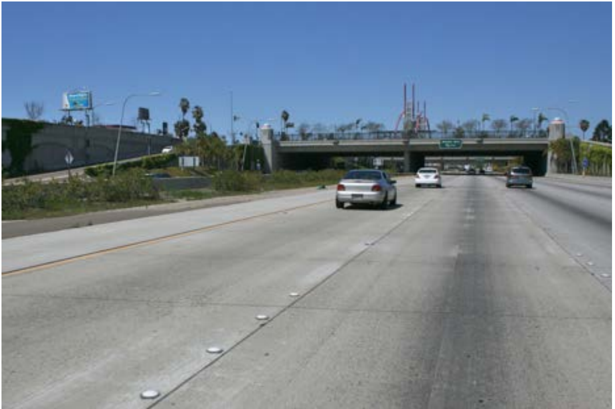
Existing Conditions: View heading northbound on SR-15 approaching El Cajon Boulevard
