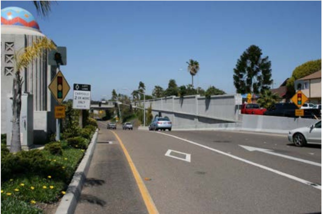
Existing Conditions: View looking north at SR-15 Northbound On-Ramp near El Cajon Boulevard
