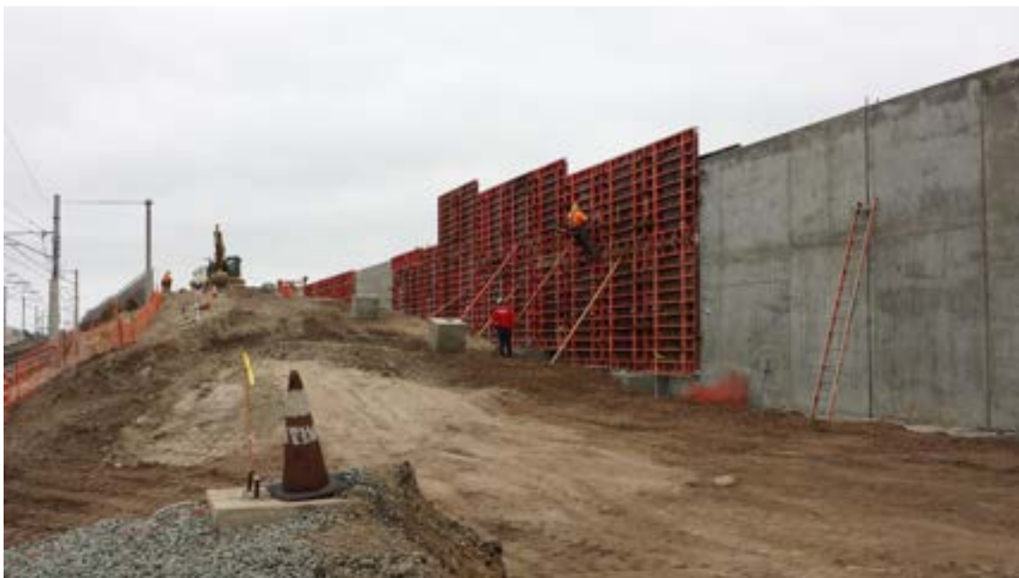
Photo 5 – Retaining Wall Construction in Progress
