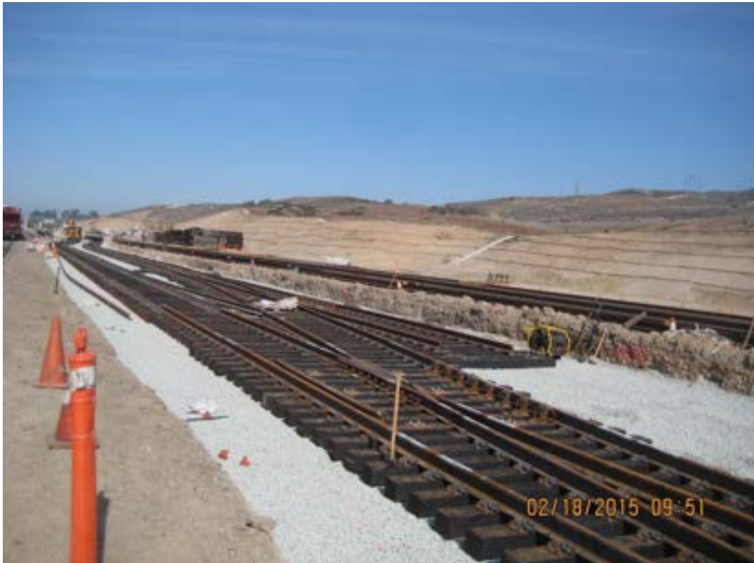
Photo 3 – Crossover Installation in Progress (February 2015)
