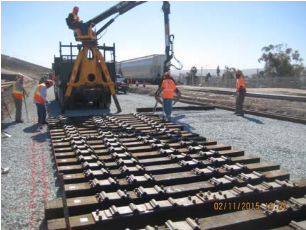
Photo 4 – Crossover Construction in Progress
