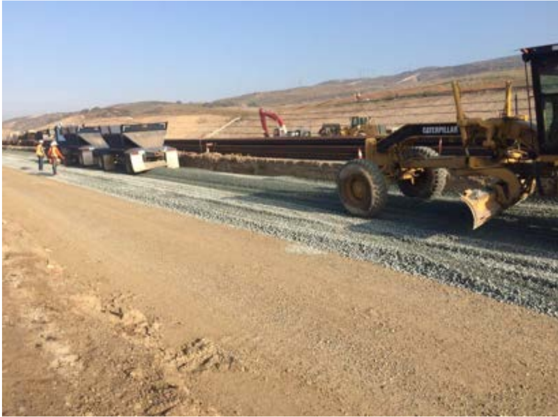
Photo 2 – Track Ballast Installation in Progress
