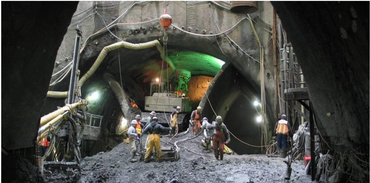
Figure 11-4. Example of Typical SEM Excavation Sequence and Final Completed Section for a Platform Tunnel
