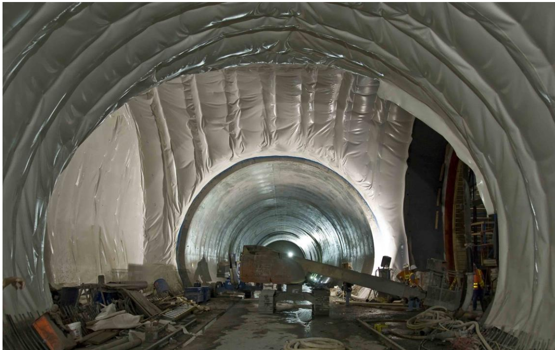
Figure 11-5. Example of Station Waterproofing
