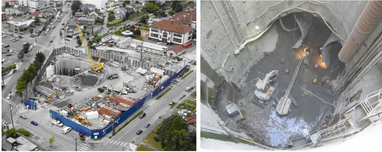
Figure 11-2. Example of Typical SEM Excavation Sequence
