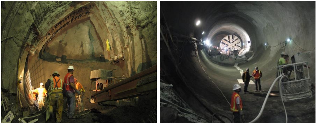
Figure 11-4. Example of Typical SEM Excavation Sequence and Final Completed Section for a Platform Tunnel
