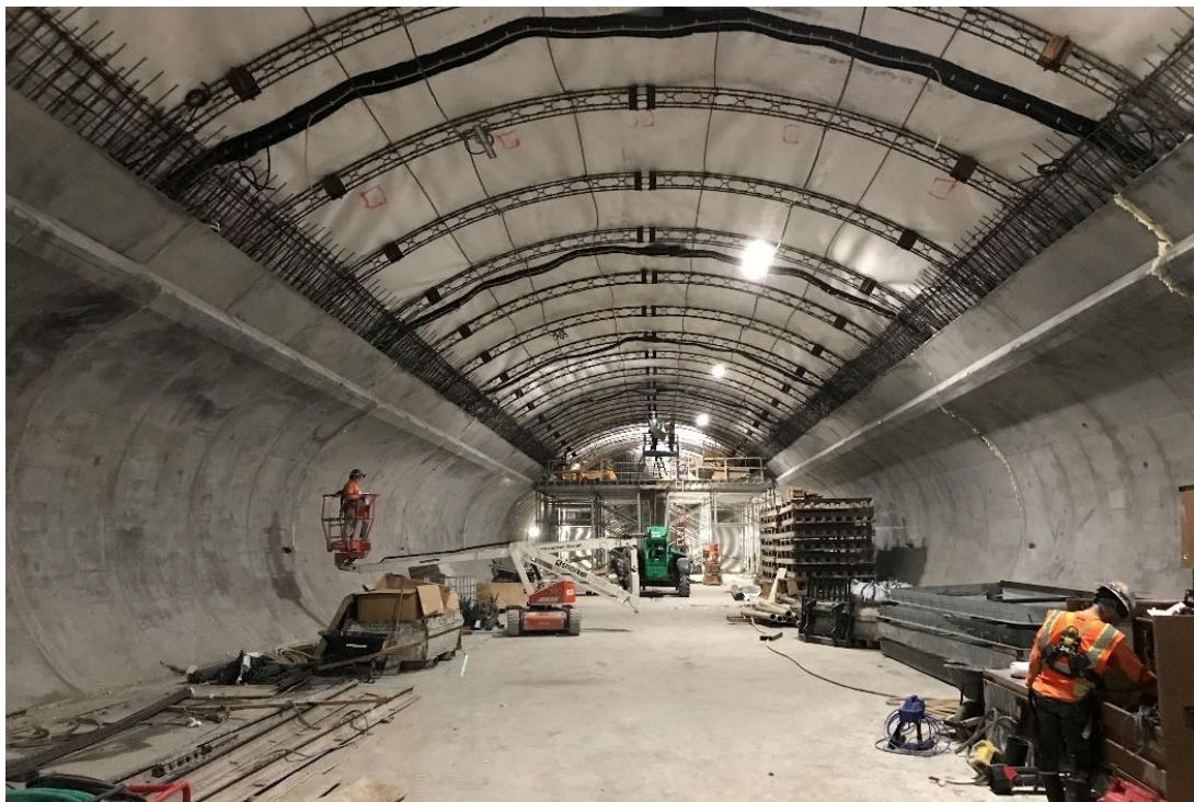
Figure 11-6. Example of the Station Final Concrete Lining
