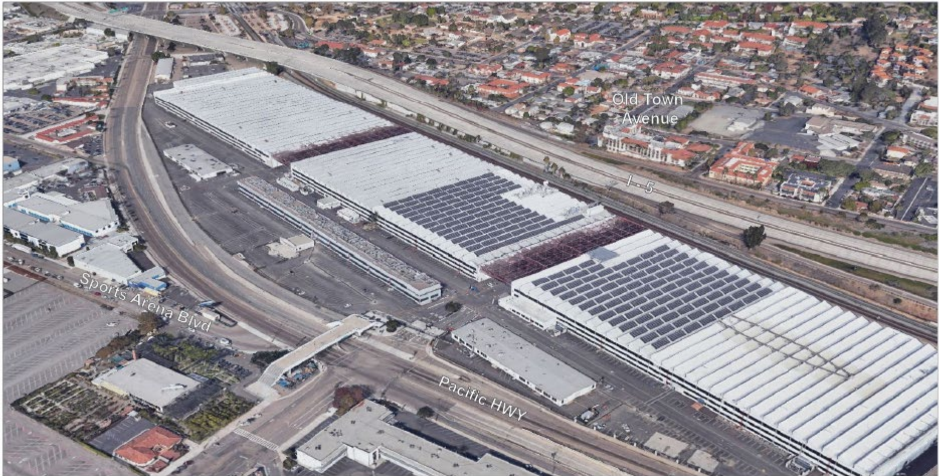
Figure A-3: Current OTC Facility Condition
