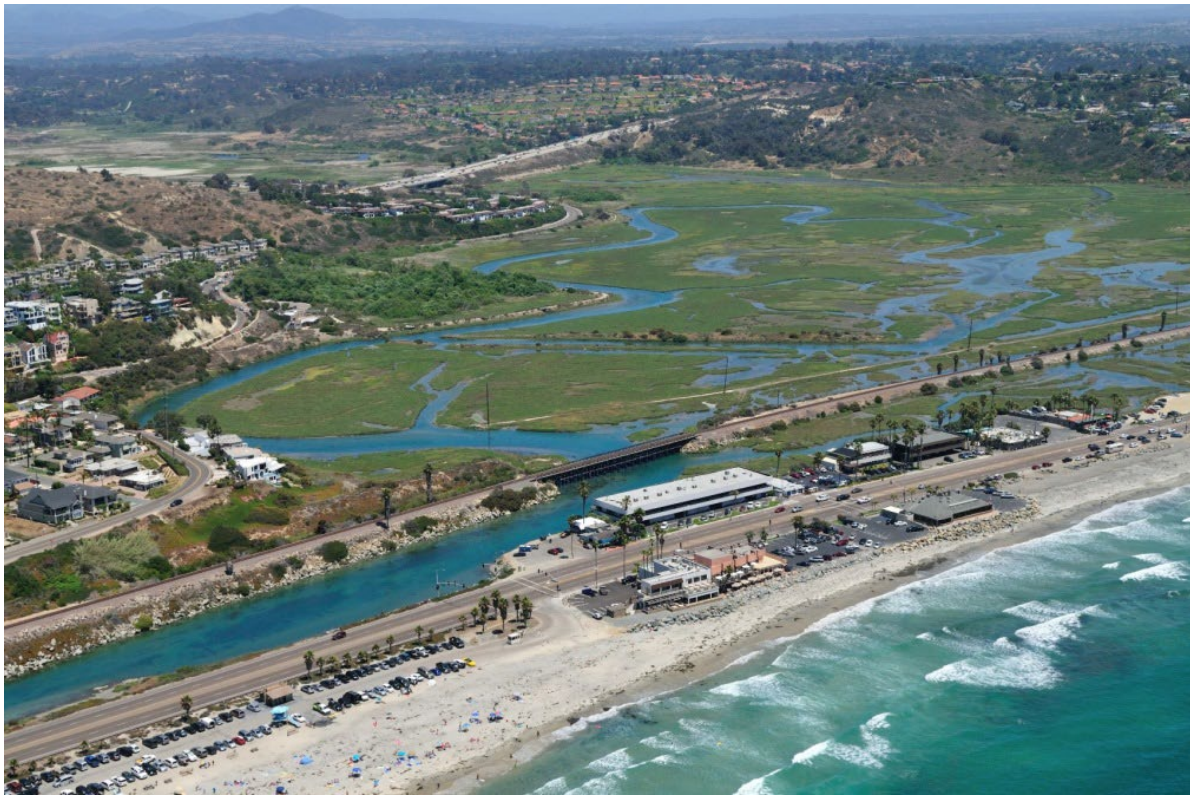
Figure 12 – San Elijo Lagoon Rail Trestle Br 240.4 substructure in Marine Severe tidal exposure (Photo Shoaff)
