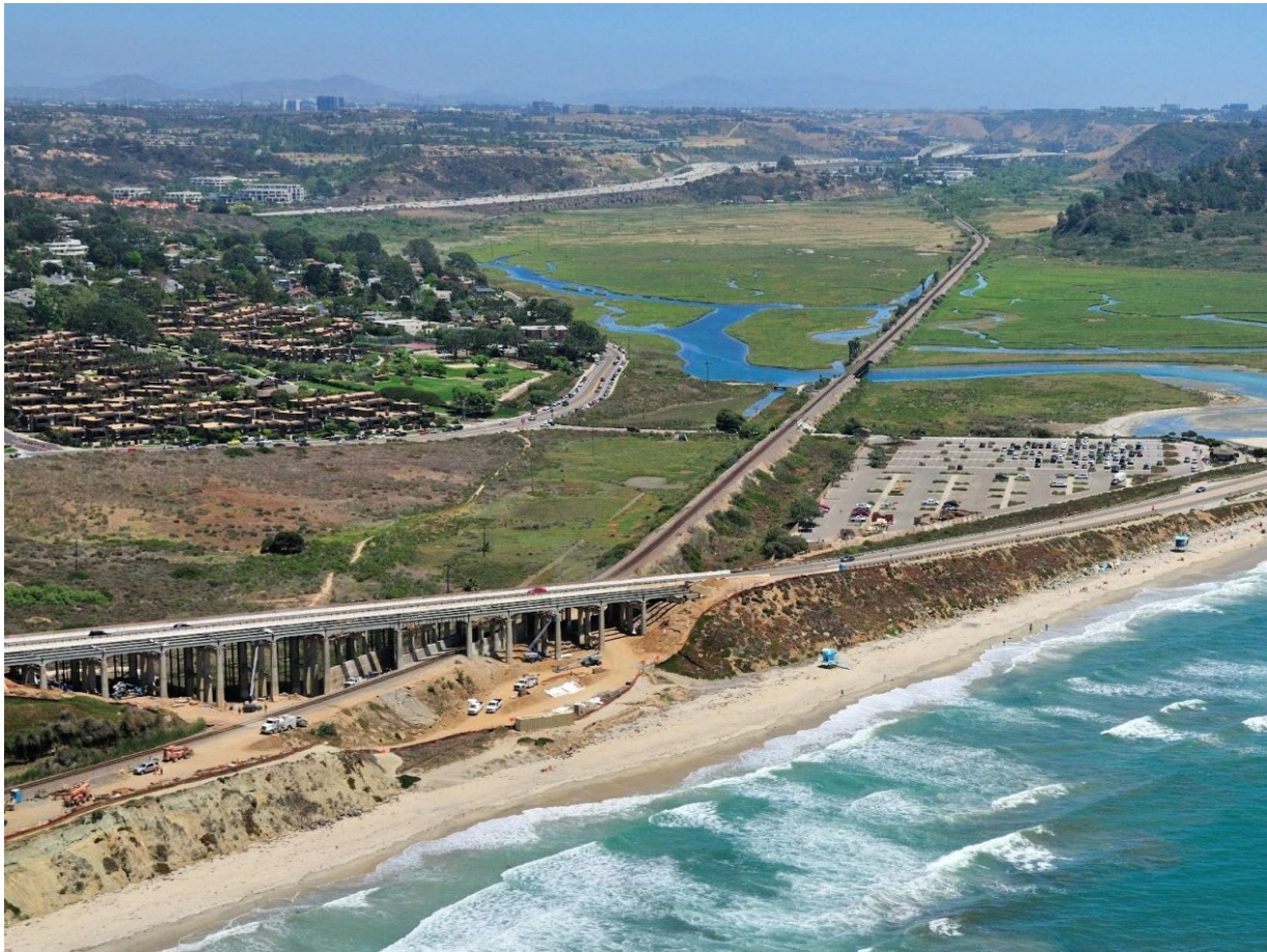
Figure 13 – Torrey Pines Overhead Br 245.7 - Marine moderate (Airborne) exposure (Photo Shoaff)
