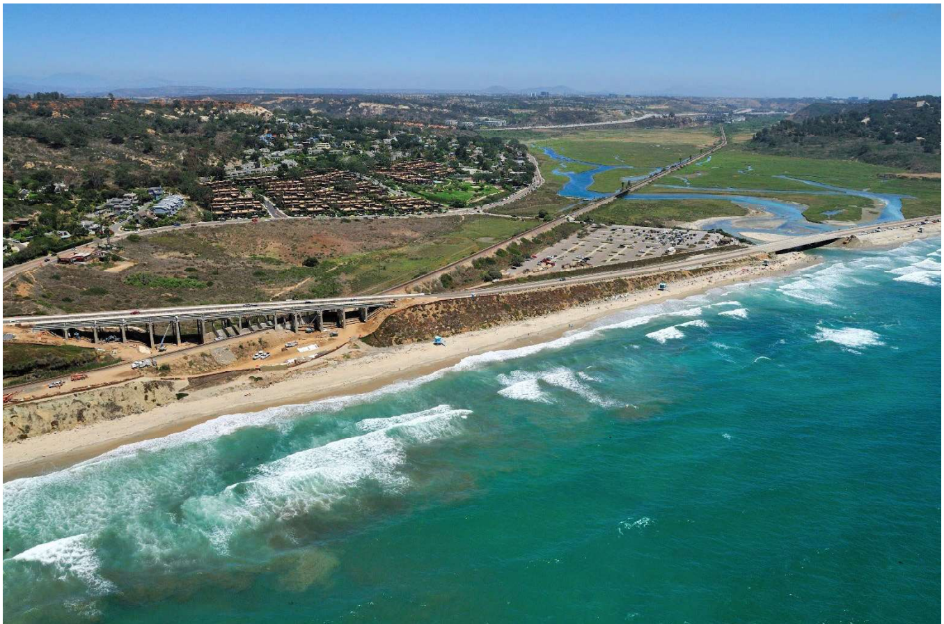
Torrey Pines overhead bridge on LOSSAN Rail Corridor
