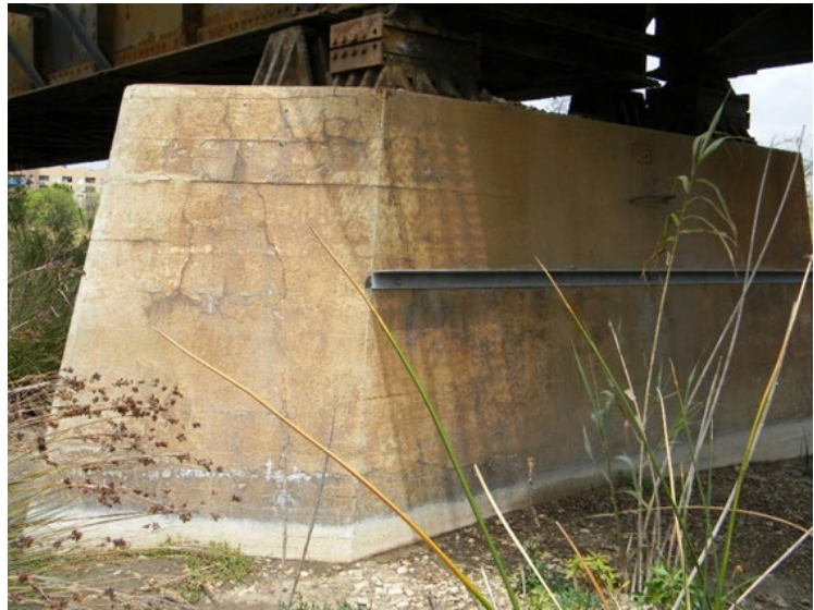
Figure 4 - Alkali aggregate reaction in Br 225.3 San Luis Rey River from 1916
