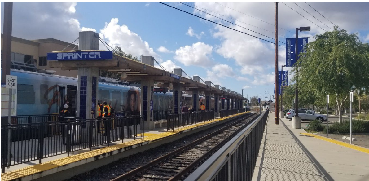
NCTD Sprinter platforms at the Escondido Transit Center in Escondido, CA.
