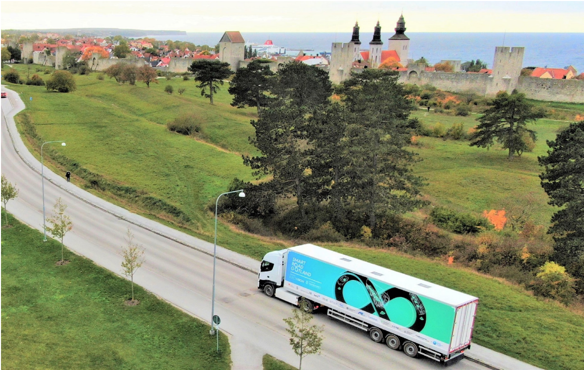
Figure 5: Public electrified road in Sweden (Source: Smartroad Gotland)
