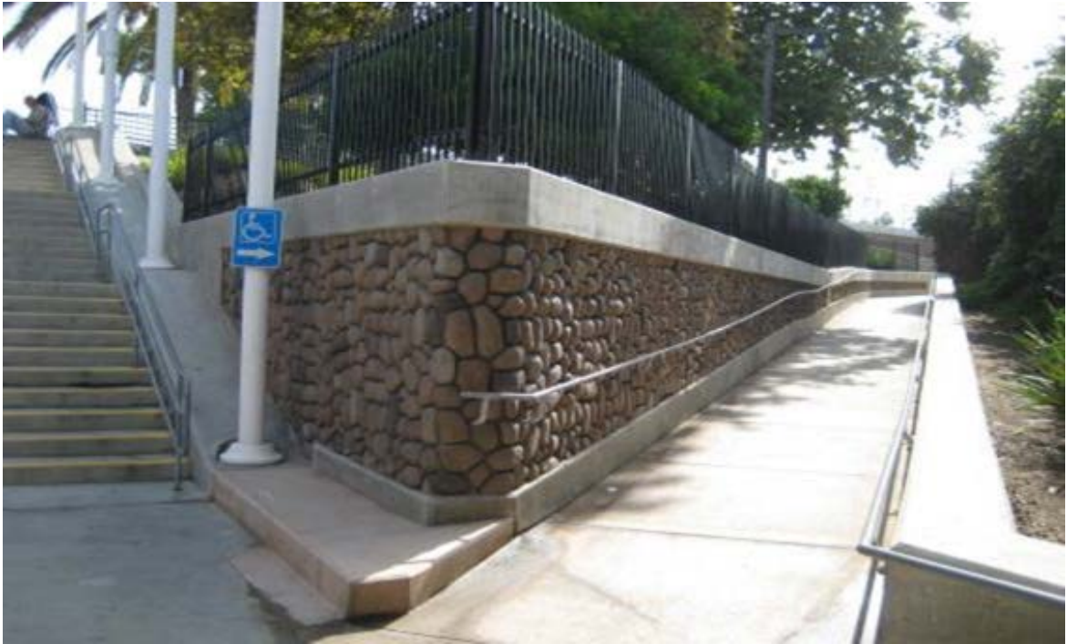
i. Old Town Undercrossing
