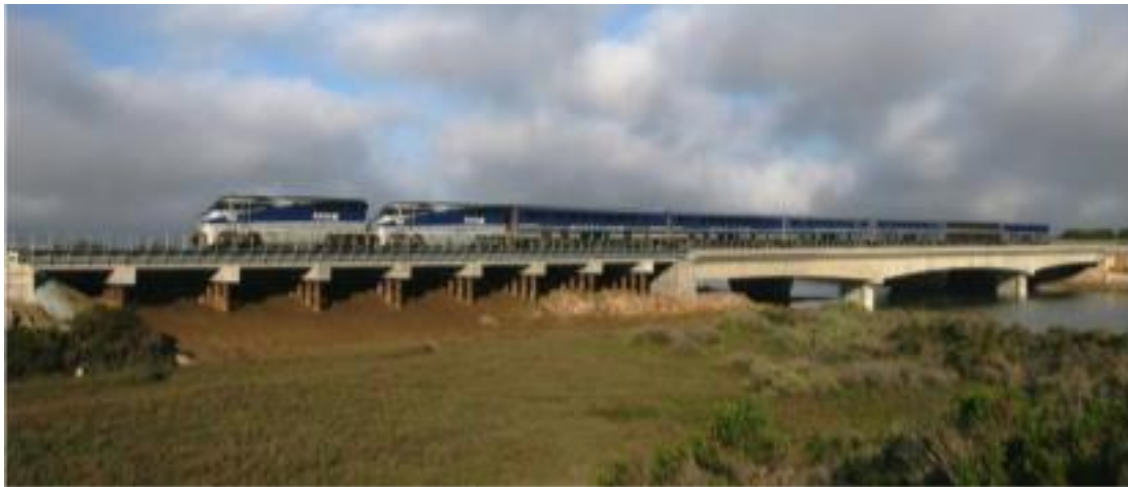
i. Santa Margarita River Bridge.
