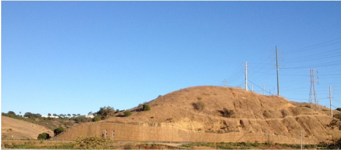
i. Sorrento to Miramar phase 1 soil nail slope treatment .
