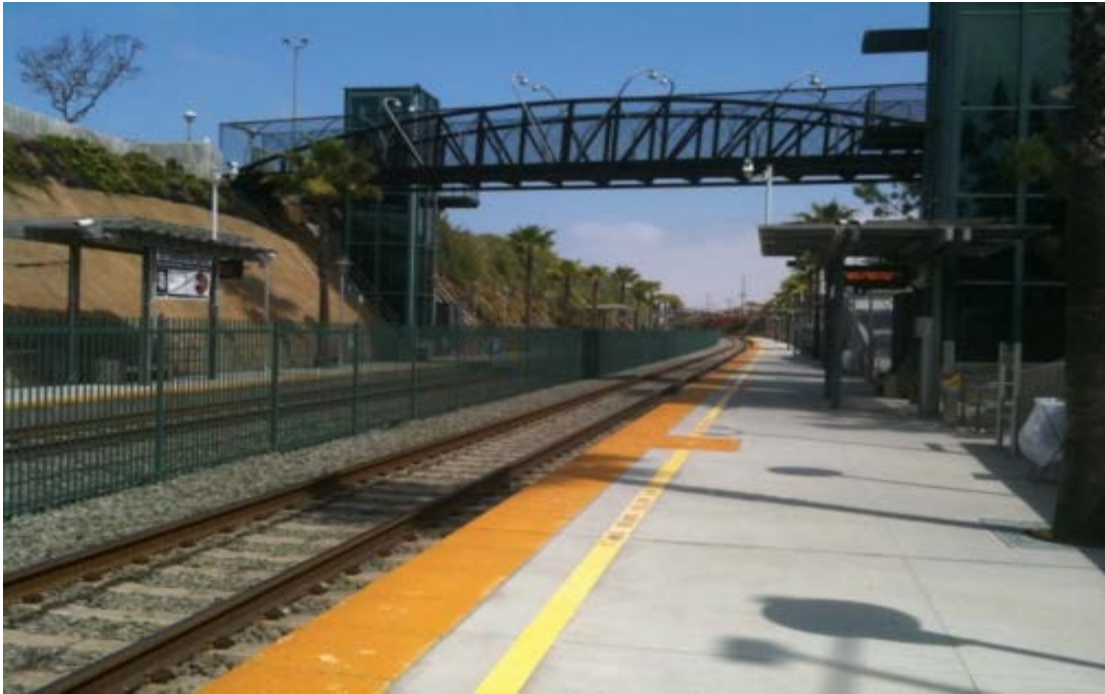
i. Solana Beach Station Bridge
