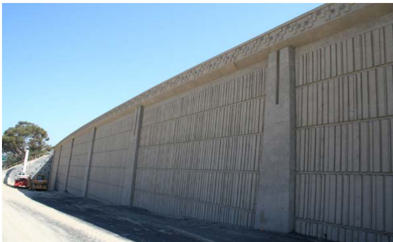
ii. Sorrento to Miramar phase 1 Retaining wall treatment.
