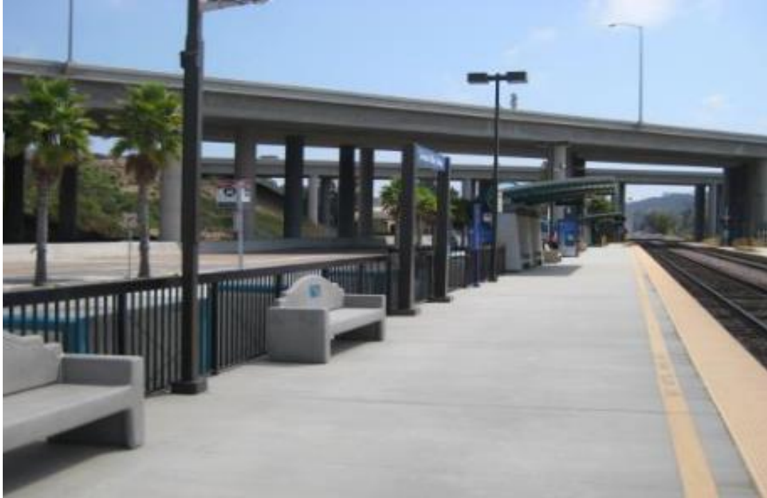
iii. Sorrento Valley Station under I-805 merge.
