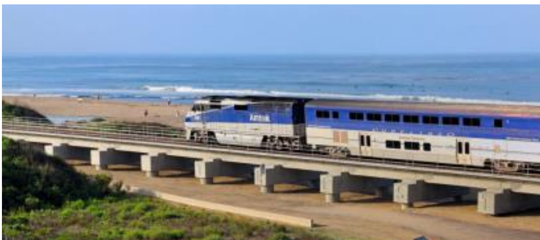
iii. Trestles Bridge over San Mateo Creek.
