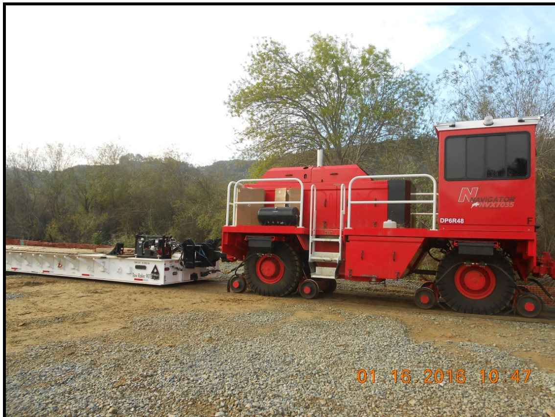
Bridge 247.7 – Photo of the TowRailer and the Shuttlewagon on the track.
