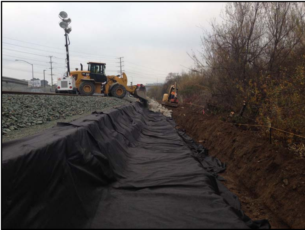
CCO #42 ADDITIONAL SLOPE PROTECTION
