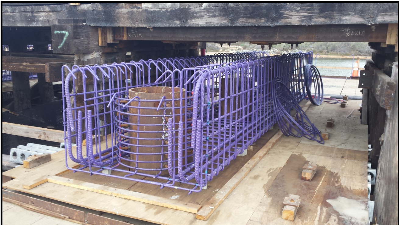
Bridge 246.1 – Forming and reinforcing of the Bent Caps has started.
