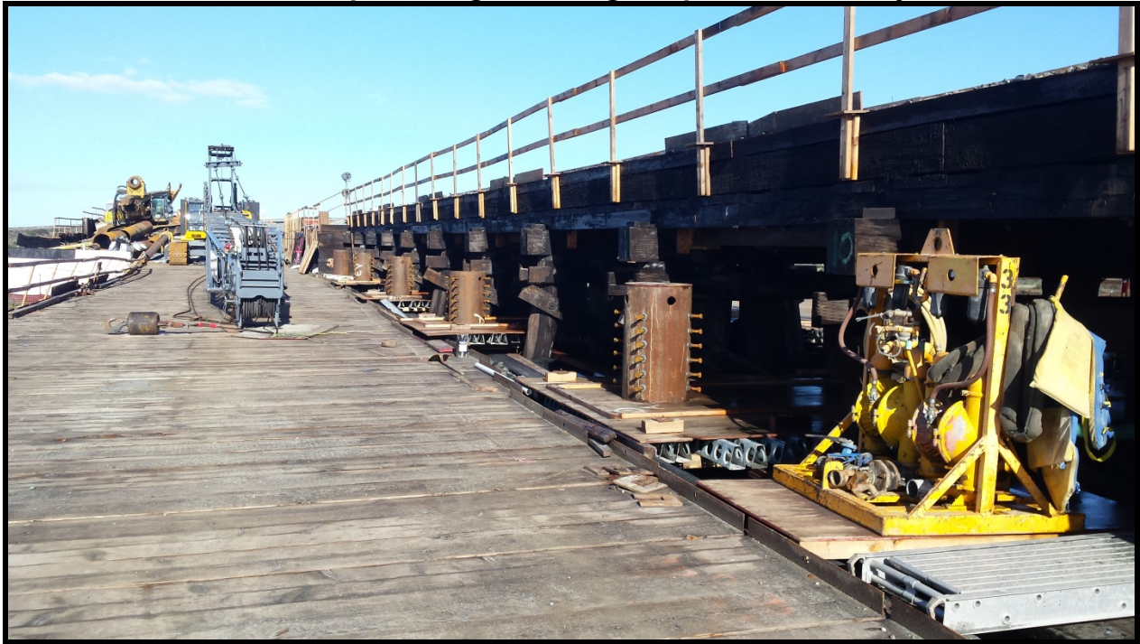
Bridge 246.1 – All 33 CISS piles at Bridge 246.1 have been installed.
