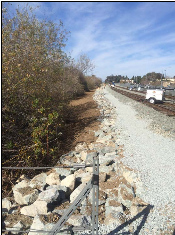
CCO #42 ADDITIONAL SLOPE PROTECTION
