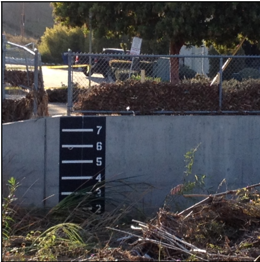
SORRENTO VALLEY FLOOD GAUGE SHOWING DEBRIS FROM HIGH WATER ON JAN 5-7, 2016
