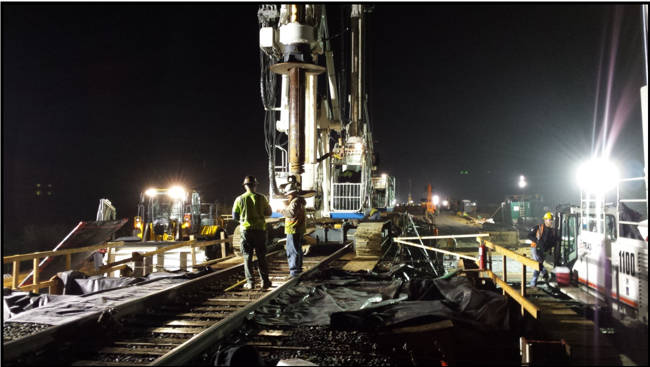
Bridge 247.1 – All 4 interior CISS piles were installed during the Jan 16-17 AWW.
