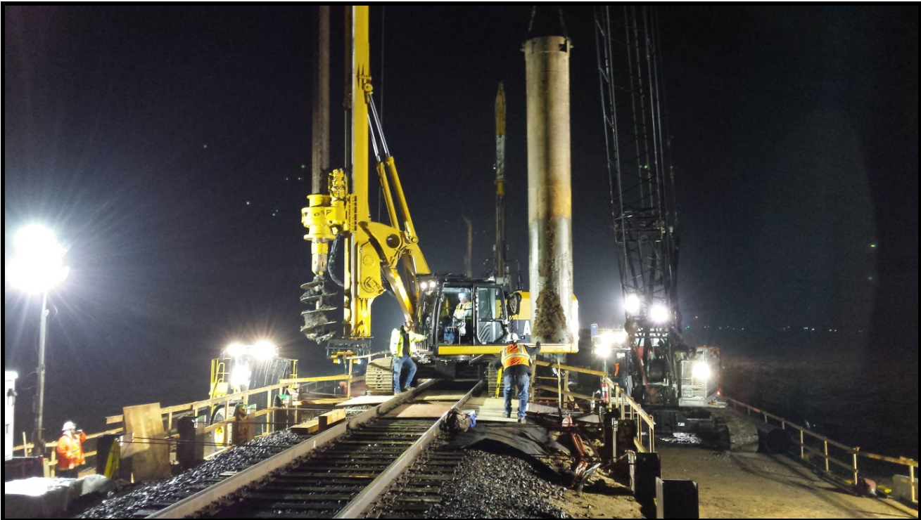
Bridge 246.9 – All 8 interior CISS piles were installed during the Jan 16-17 AWW
