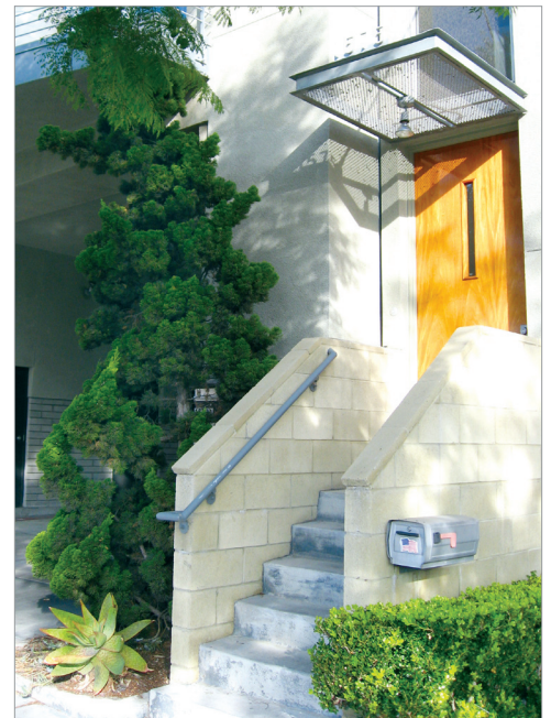
Entrances to new housing face the street.
