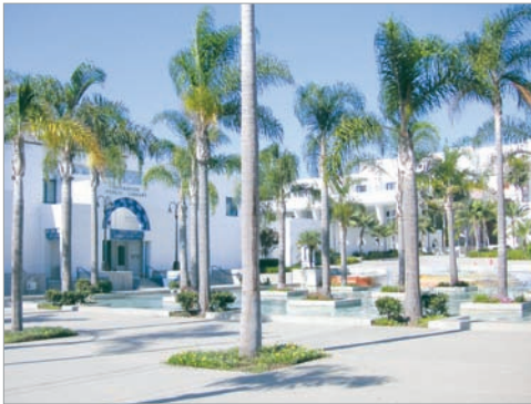
A pool and plaza mark this entrance to the Oceanside Public Library.
