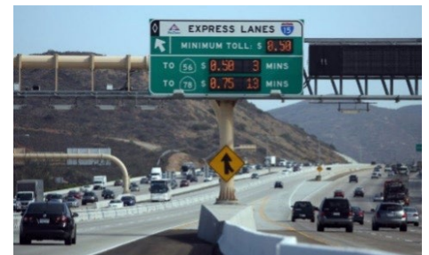
The I-15 Express Lanes in San Diego are an example of Managed Lanes (Source: Union Tribune)
