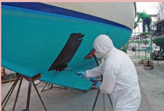
Marine coatings are frequently used in San Diego County
