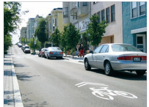
A shared lane marking in San Francisco, California, denotes a travel lane shared by bicycles and cars.
