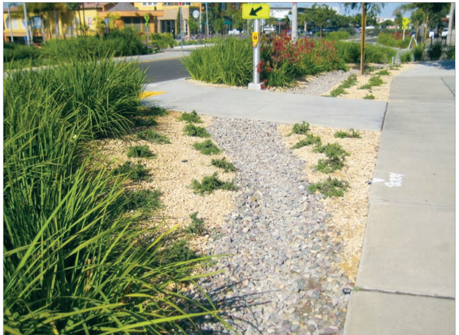
Permeable surfaces, such as this landscaped bulbout in La Jolla, reduce stormwater runoff.
