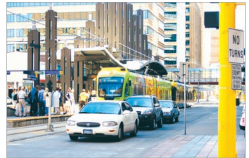
LRT lanes can be physically separated from vehicle lanes to prevent conflicts, as shown in this example from Minneapolis, Minnesota.
