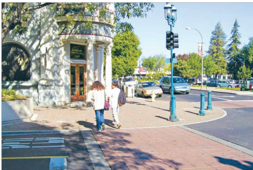
This intersection in Redwood City, California, includes highly visible crosswalks as well as bollards that protect pedestrians from turning vehicles.
