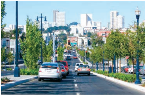
Multiway boulevards, such as this portion of Octavia Boulevard in San Francisco, California, provide room for through and local traffic, as well as space for bicyclists and pedestrians.
