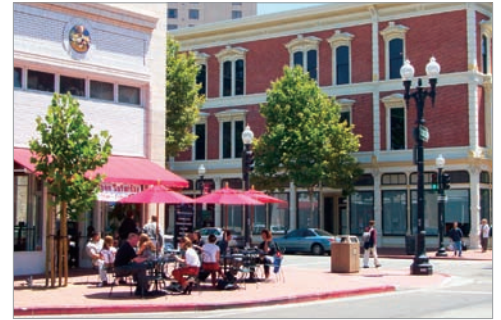
Bulbouts such as this one in Oakland, California, narrow streets and provide space for pedestrian amenities.
