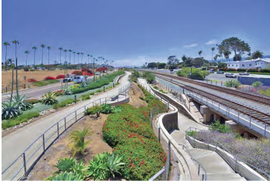
Figure 3.7: Chesterfield Drive to Santa Fe Drive Undercrossing Segment
