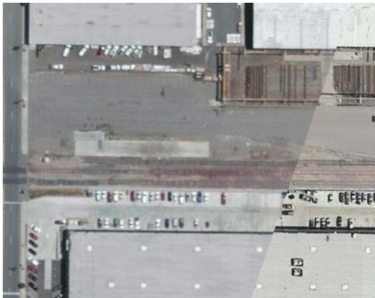
Figure E.29: National City Team Track
