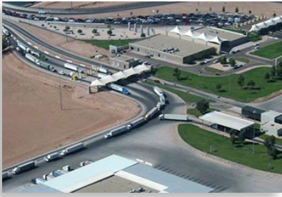
Northbound Calexico East border crossing.
